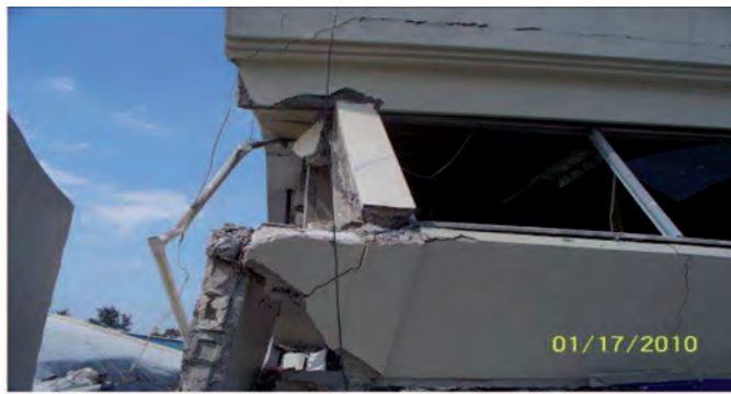
(b) A detail of (a), notice the inadequate reinforcement
