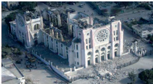
(b) Aerial view from N-W side. All main walls of the Cathedral remain intact, vertically.
