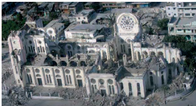
(a) Aerial view from S-E. The roof collapsed within the ground plan of the Port-au-Prince Cathedral.
