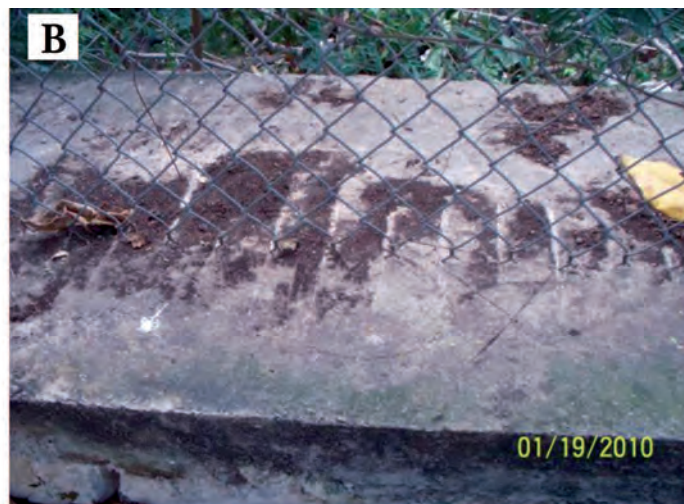
(b) Details A of the observed imprints – light scratches, by the lower wires on the steel net on the concrete base. The direction of the motion is NE-SW.
