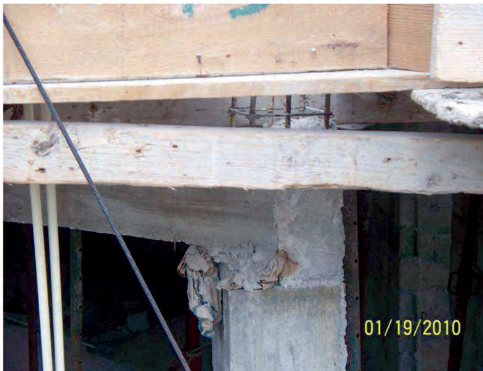
(b) A detail of a column to beam joint of the framing system shown in (a).
