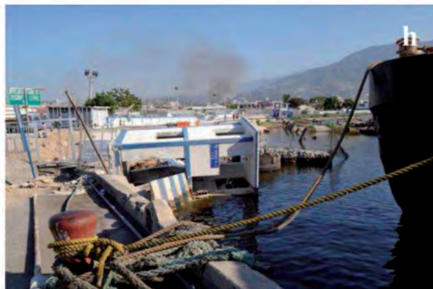
Fig. 3a-h. Extensive liquefactions and lateral spreading phenomena caused significant damages in the port facilities of Port-au-Prince. Marine transportations and shipping were interrupted during the initial period after the main shock.
