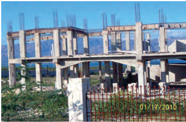
Fig. 12. A reinforced concrete framing system was ready for concreting before the earthquake as found after it. Total lack of any stiffening element. Note the beam at the center of ground floor with the triangle strut was added after the concreting of the floor.
