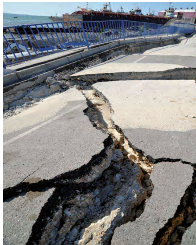
Fig. 5. Port-au-Prince port area. The ejected material could form a continuous surface if the broken pieces are assembled together like in a puzzle. This shows that sand and water ejections started before the actual liquefaction and the lateral spreading phenomenon took place.
