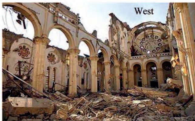
(f) Internal view of the Cathedral of Port-au-Prince. The roof collapsed within the plan of the church.
