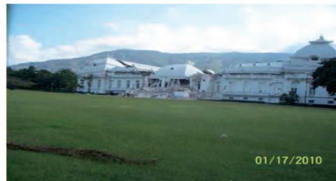
(f) The Presidential Palace. An almost symmetrical vertical collapse of the upper level.
