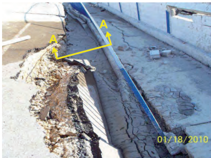
(a) General view of the trench with ridge of liquefied material inside it.
