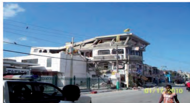
(d) Typical collapse of a multi-storied buildings with reinforced concrete framework.
