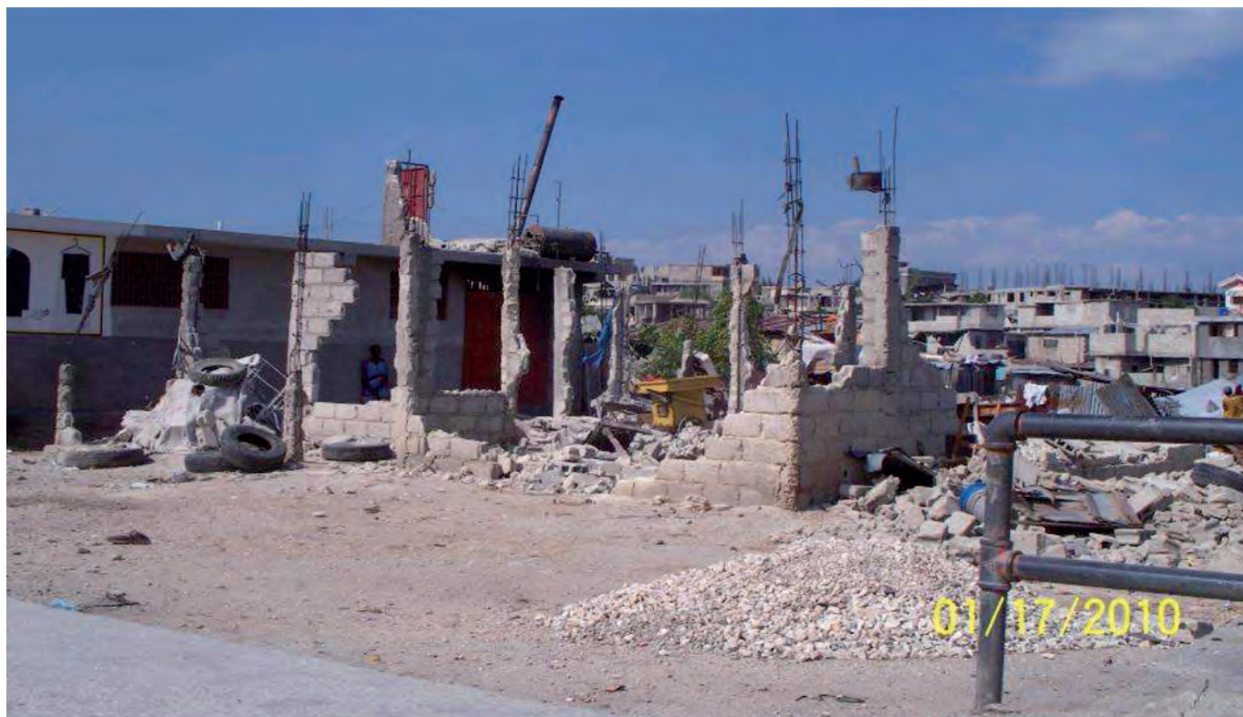
Fig. 10. Typical view of the way of self constructing of low income masonry buildings.
