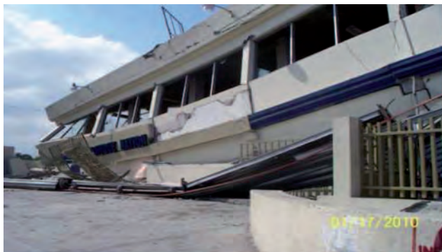
(a) Typical collapse of a contemporary building with reinforced concrete framework.
