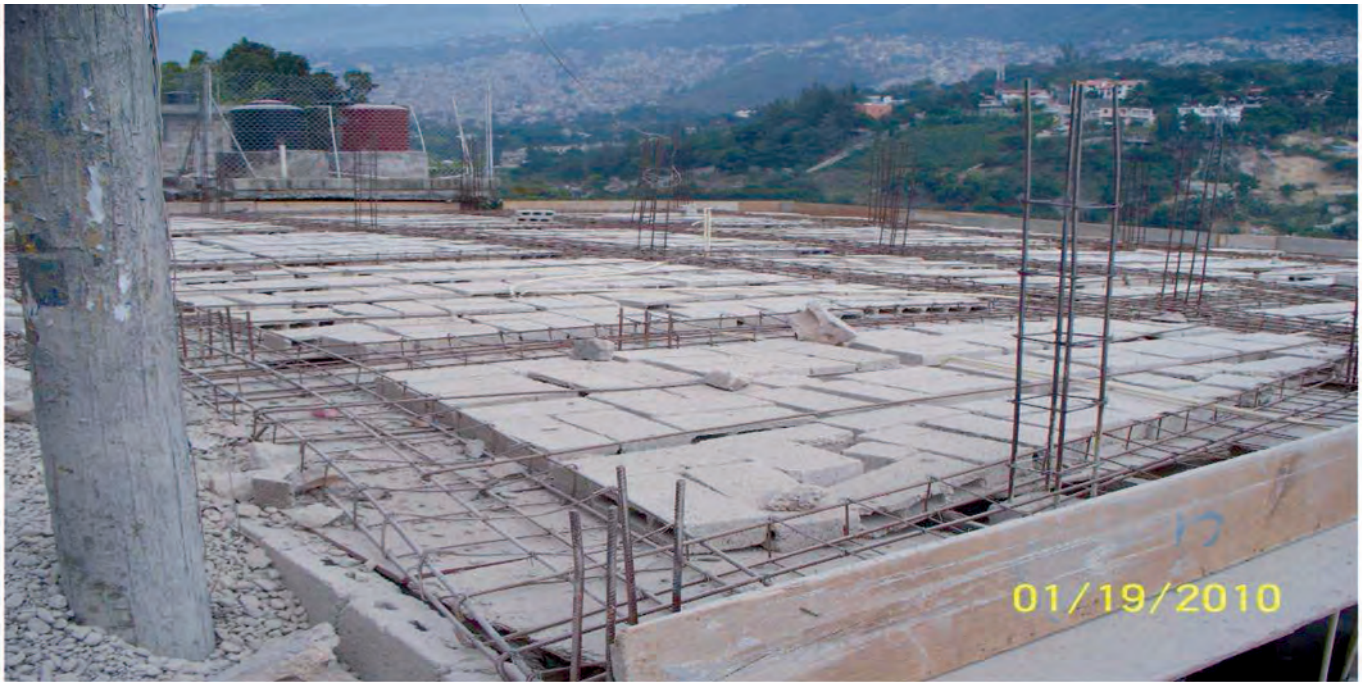
(a) Flat slab construction of the third floor. Inadequate reinforcement of small diameters and at large distances. Small dimensions of columns. Absence of any shear wall.
