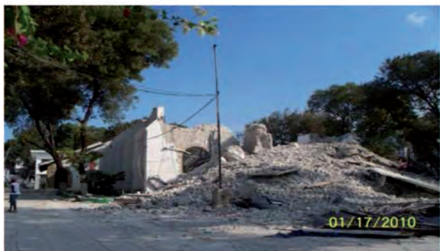
(e) The arch-like lintels over the windows survived.
