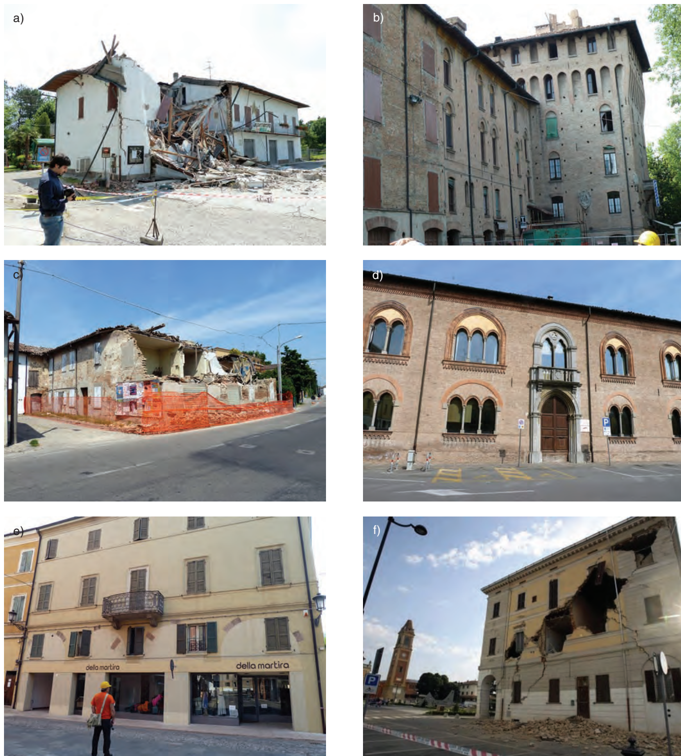
Fig. 36. A selection of representative damage incurred in masonry buildings as well as undamaged buildings. Each one of those deserves a special in depth investigation.
