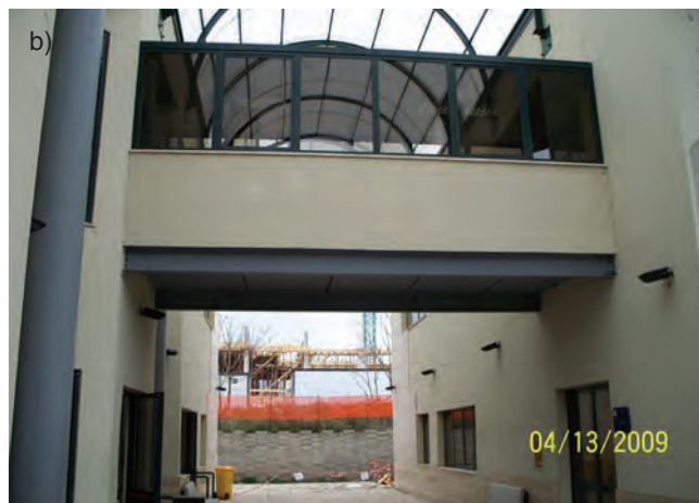
Fig. 19. The differential horizontal motion between neighboring structures is usually expressed by some damage in the bridging structure and the connecting parts; a) in the ceramic factory in Sant' Agostino and b) in the University of L'Aquila after the 2009 earthquake. At both cases not any sign of differential horizontal motion was noticed.
