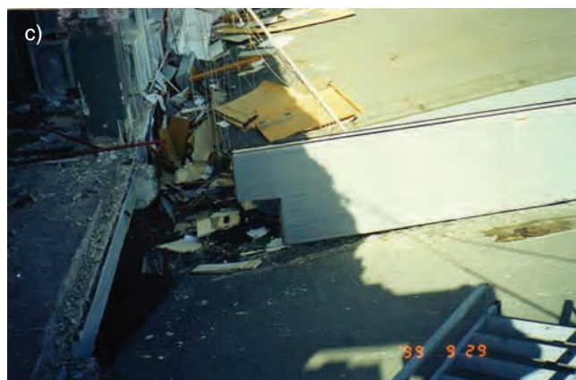
Fig. 31. a) Due to the vertical seismic component, the beam is jumping up and down on its supports if it is not sufficiently anchored; b) the corbel or the beam, or both are broken. In this case a vertical bolt is provided but it was too short and the beam jumped over; c) if there is a horizontal motion too, the results are worsened.
