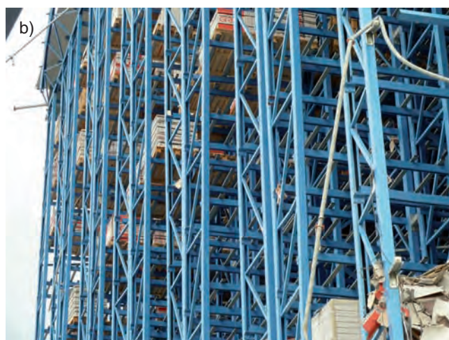
Fig. 18. a) A part of the ceramic warehouse in Sant'Agostino totally collapsed; b) This part of the same warehouse did not move. This can be very well justified by the relative position of the stored material to the steel members of the racks, which is in all positions the same. It must be taken under consideration that the positioning of the stored materials is computerized.
