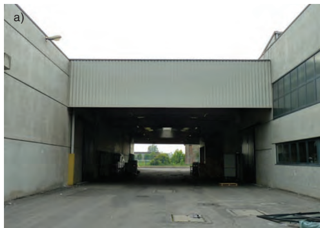
Fig. 19. The differential horizontal motion between neighboring structures is usually expressed by some damage in the bridging structure and the connecting parts; a) in the ceramic factory in Sant' Agostino and b) in the University of L'Aquila after the 2009 earthquake. At both cases not any sign of differential horizontal motion was noticed.
