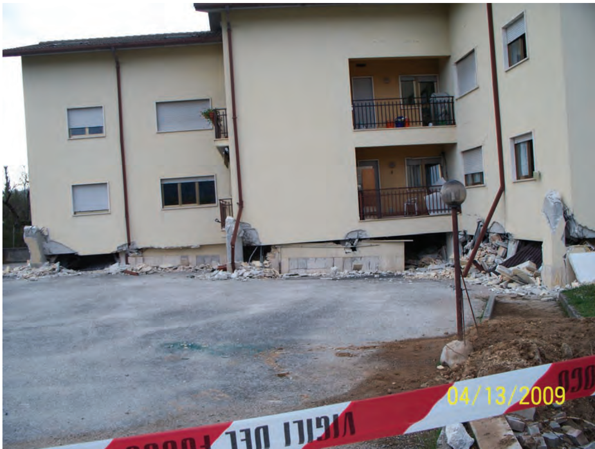
Fig. 24. During the L'Aquila, 2009 earthquake all perimetric columns at the base of the structure were displaced outwards, the building sat down almost vertically, while most of the glass panels remained unbroken, and almost no other damage was optically observed from the outside.
