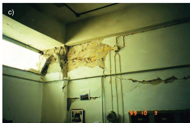
Fig. 29. "Short column", under a vertically propagated body wave action. The braking plane is perpendicular to the plane of the concrete wall and the respective beam. The adjacent window glass panel is unbroken. Not any significant residual vertical shortening is noticed. In c) the presence of a masonry wall perpendicular to the plane of the concrete wall did not prevent the break of the "short column".
