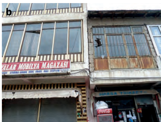
Fig. 21a, b. No evident horizontal motion, or breaking of glass panels, or pounding between adjacent buildings was observed.
