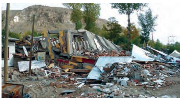
Fig. 26a, b. An other technically interesting collapse: a) In the fore-ground is the roof and the roofing corrugated iron-sheet; b) The top is the back column. The other columns are shaken off. Note that a flat-slab construction system does not allow any space for protection during collapse. The owner was describing that during the main shock he was staying on the ground. He felt two extremely violent upwards jolts, the one followed by the second making him to jump-up. At that time the building was jumping-up too. It was balancing, at the first cycle it stood on the front columns in parallel to the street. Next, the building stood on the back columns and then in the front ones with a stronger stroke when it toppled over.
