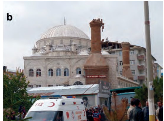
Fig. 18a, b. Most of the mosques with their minarets weathered the main shock without any damage. In a limited number of cases parts of minarets toppled.
