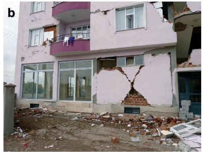
Fig. 28a, b. Note that the glass panels are intact while the walls are damaged especially at the lower levels. This is the case for almost the majority of the damaged-not collapsed multi-storeyed buildings, in Ercis city.
