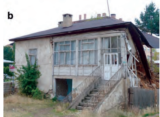
Fig. 16a, b. This manner of damage of simple houses indicates the dominance of vertical seismic component.
