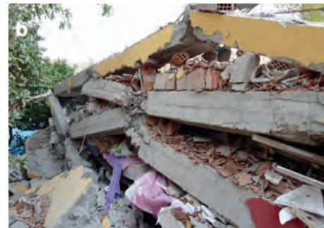
Fig. 26a, b. An other technically interesting collapse: a) In the fore-ground is the roof and the roofing corrugated iron-sheet; b) The top is the back column. The other columns are shaken off. Note that a flat-slab construction system does not allow any space for protection during collapse. The owner was describing that during the main shock he was staying on the ground. He felt two extremely violent upwards jolts, the one followed by the second making him to jump-up. At that time the building was jumping-up too. It was balancing, at the first cycle it stood on the front columns in parallel to the street. Next, the building stood on the back columns and then in the front ones with a stronger stroke when it toppled over.
