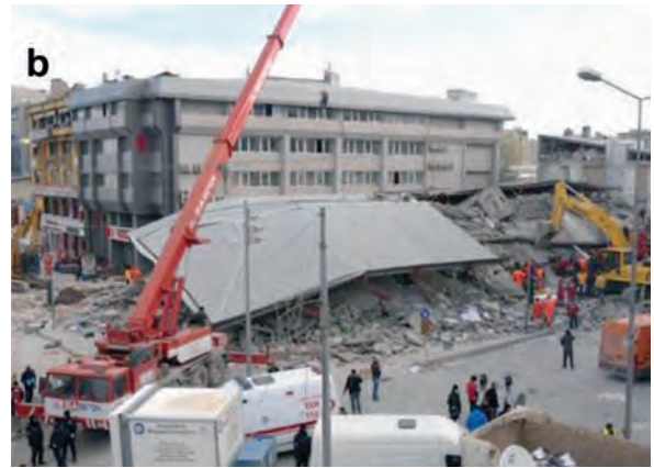
Fig. 30. a) The free standing Bayram Hotel before the earthquake and after the addition of a floor with a light weight roof. b) The collapsed roof is covering the plan, of the collapsed building in a parallel way to the pavements.
