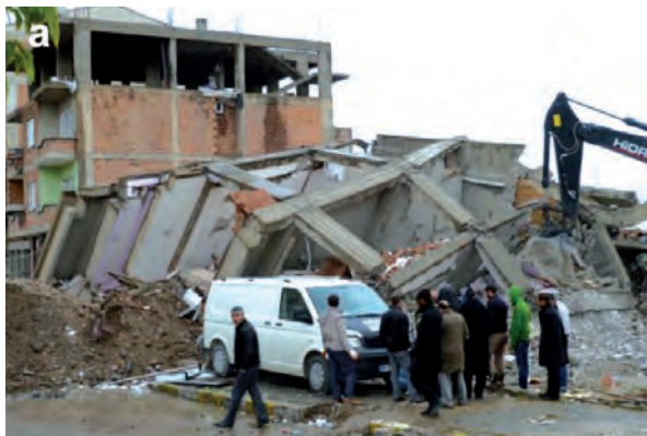
Fig. 25a, b. A technically interesting collapse. The reinforcement detailing is acceptable. Perhaps the concrete quality might have a problem or the concreting.
