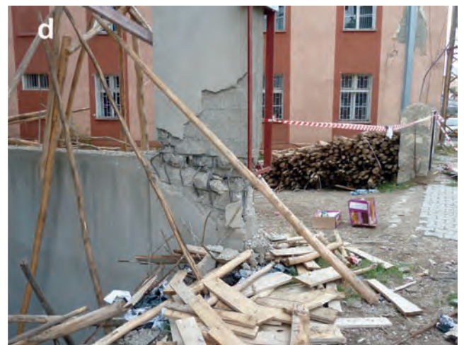
Fig. 29a-d. A just erected building with acceptable reinforcement detailing. The majority of the columns in the ground floor suffered mainly compression damages. There are no noticeable horizontal displacements.
