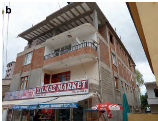
Fig. 20a, b. Usually, one or two storeys are added at the top and the balconies are externally closed with masonry partitions.
