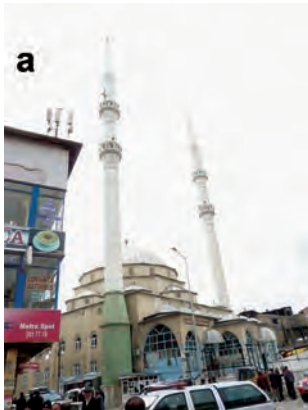
Fig. 18a, b. Most of the mosques with their minarets weathered the main shock without any damage. In a limited number of cases parts of minarets toppled.
