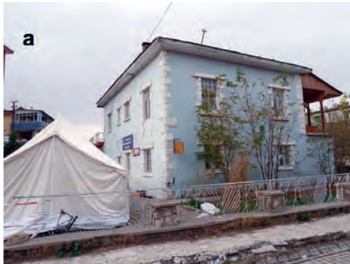
Fig. 17a, b. Traditional masonry buildings survived the main shock with minor or no damage.
