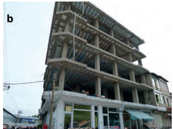
Fig. 19a, b. Flexible buildings with rather large openings and without shear walls, as well as those with a one way flat-slab construction system are prevalent in new structures.
