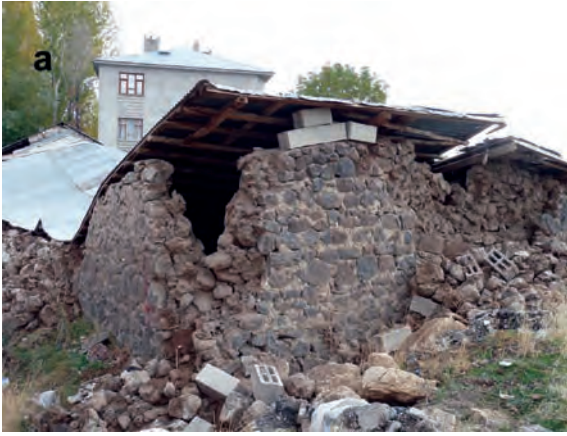
Fig. 16a, b. This manner of damage of simple houses indicates the dominance of vertical seismic component.
