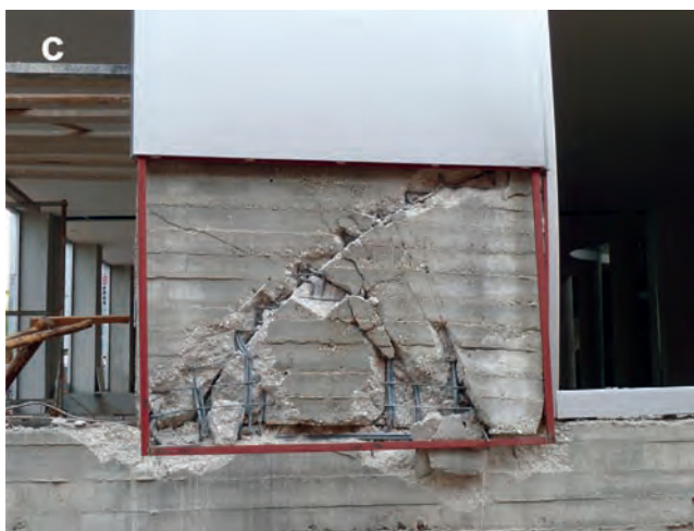
Fig. 29a-d. A just erected building with acceptable reinforcement detailing. The majority of the columns in the ground floor suffered mainly compression damages. There are no noticeable horizontal displacements.
