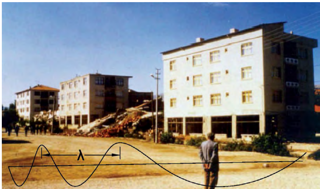
Figure 6: Rhythmic destruction. Two out of five quite similar structures founded on the same soil conditions and constructed by the same constructor totally collapsed after the Dinar, Turkey earthquake of 1995, [14].
