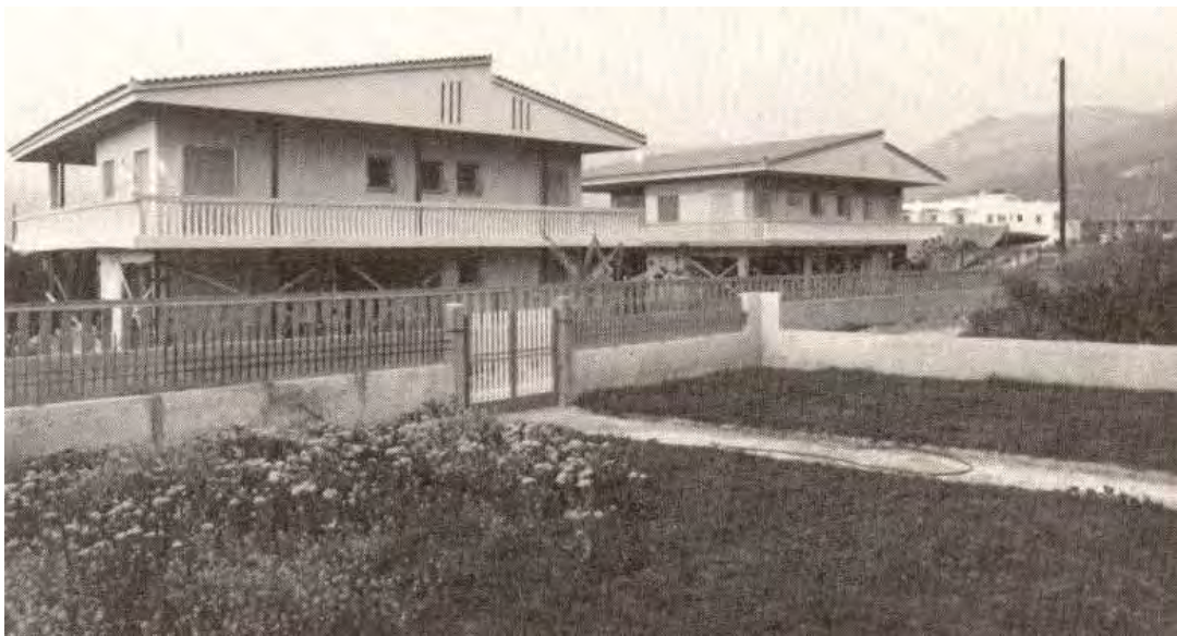
Figure 5: Rhythmic destruction. Three quite similar buildings in close distance to each other, on the same soil conditions, present a different response after the Corinthos, Central Greece earthquakes of 1981. The damage increases from the left hand side of the picture to the right hand side. The third building totally collapsed, [13].
